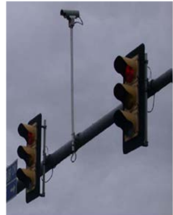
Mast Arm Mounting with Pelco Bracket
