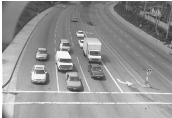
Acceptable Camera Alignment
