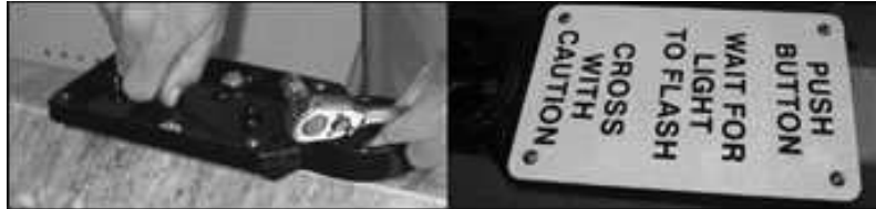
Figure 6-5: Push-button plate (left) and sign (right)
